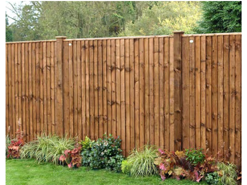
Timber closeboard fence for boundary between houses
