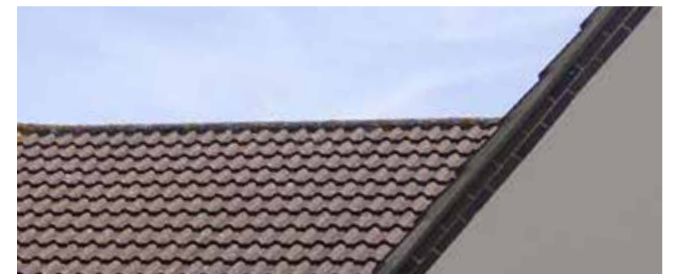
4 Roof detail along Whitmore Road
