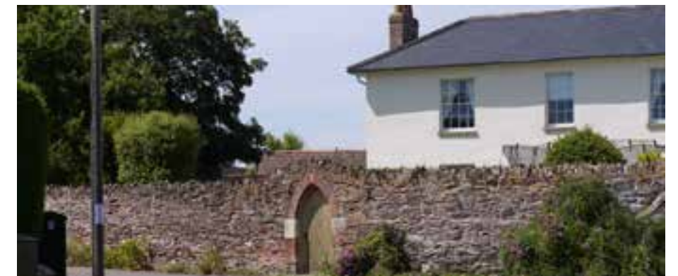
3 Feature stone wall along Rectory Road
