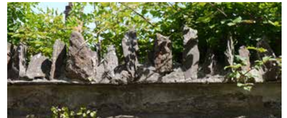
2 Stone wall detail along Rectory Road
