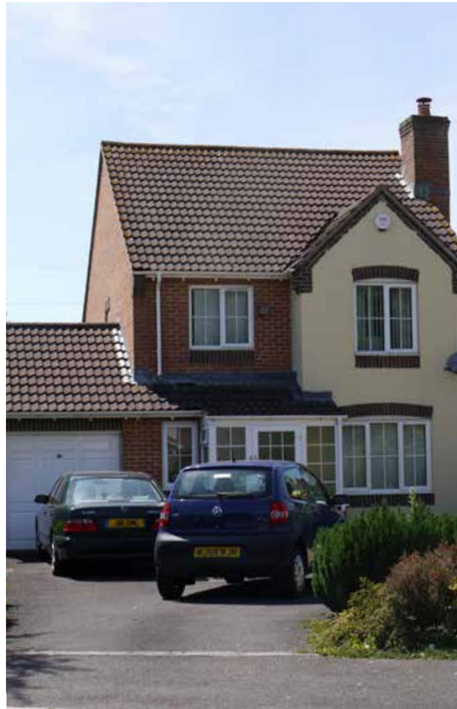
1 Typical house along Showell Park
