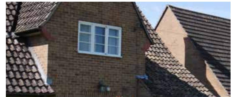
2 Gable elevation along Whitmore Road
