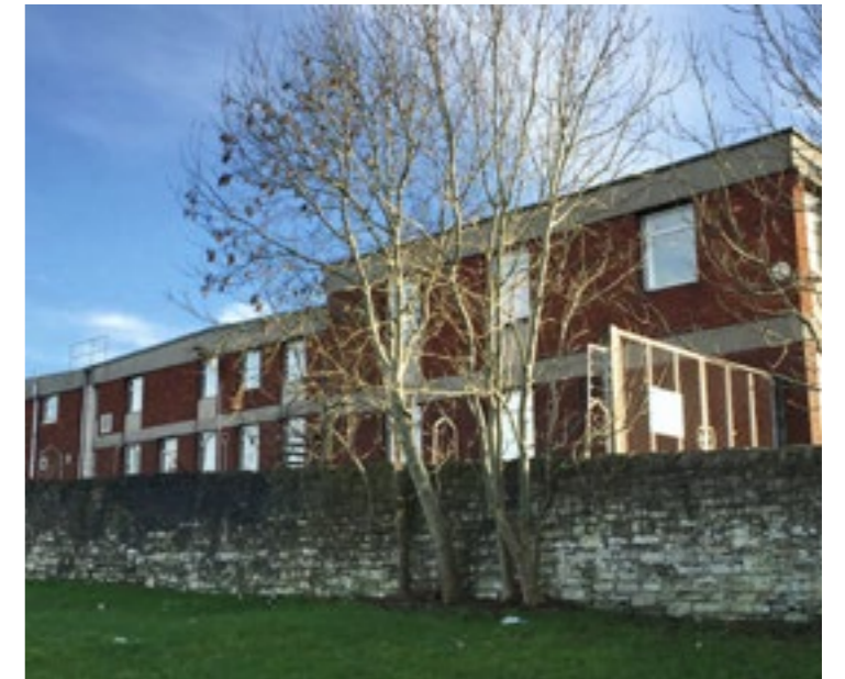
Existing stone wall as seen from the park
