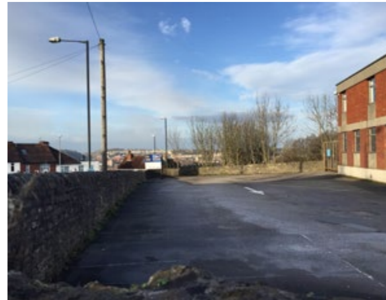
Existing stone wall as seen from within site
