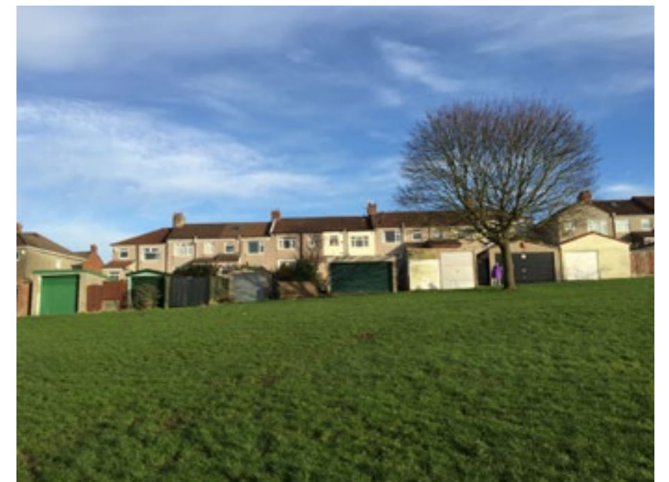
3. Existing Garages Facing Park
