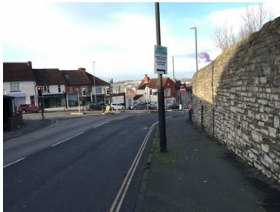
5. Existing Stone Wall on the Boundary of the Site
