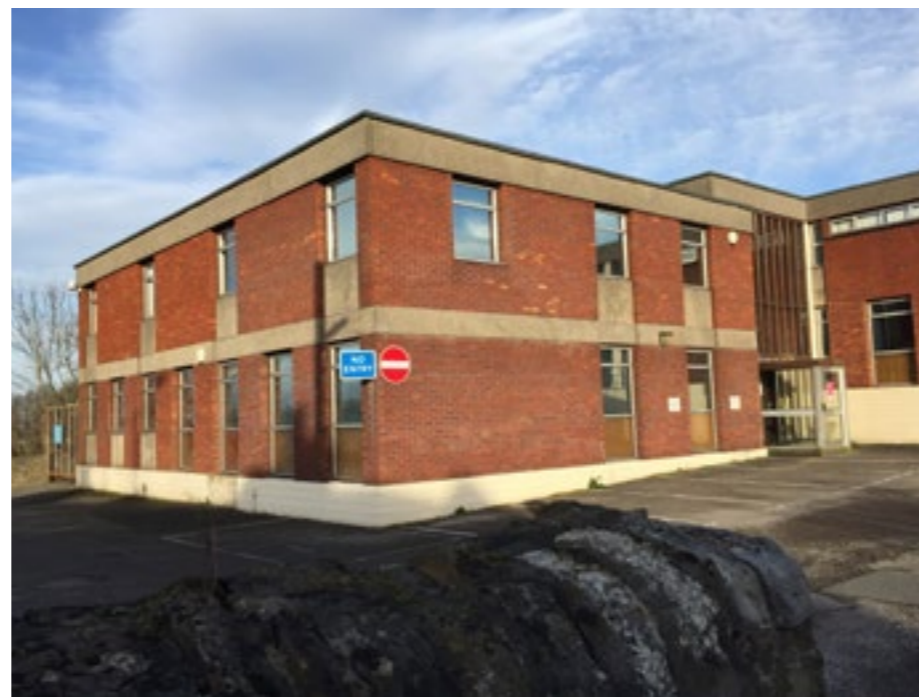
6. Existing Buildings on Site
