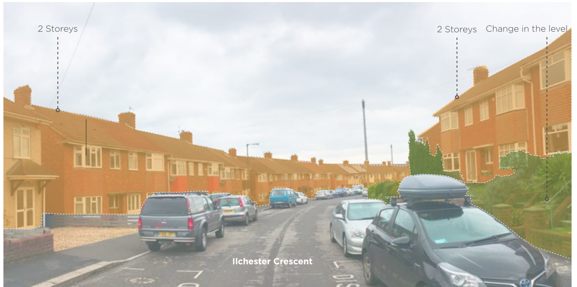
1. Housing along northern end of Ilchester Crescent where a change in level occurs across the road
