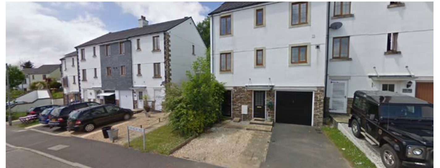
6 Eaves typically run parallel to street
