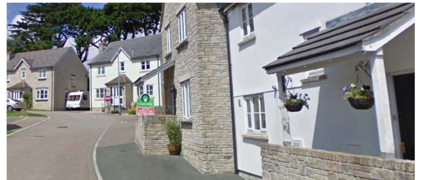
7 Street elevations are typically stone, render or weatherboarding
