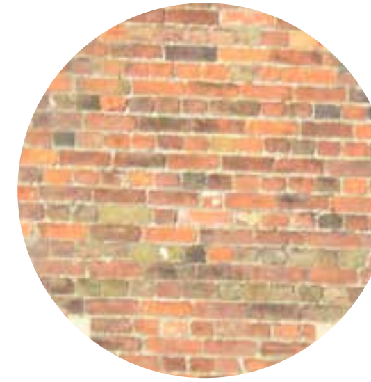
1. Existing Brick Buildings on Site
