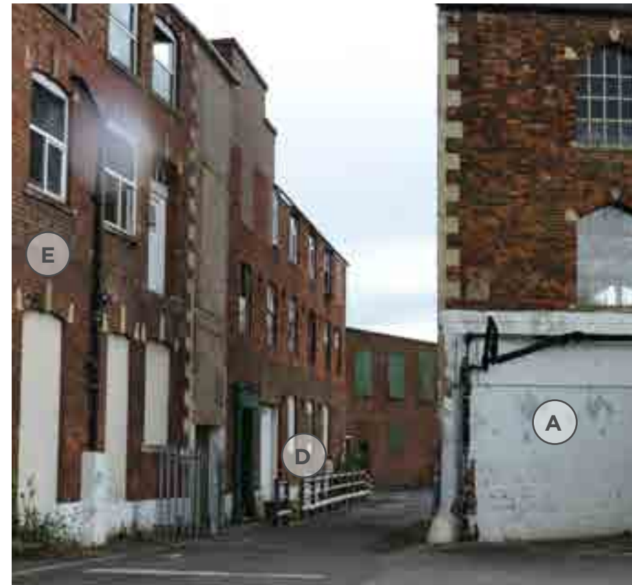
View of the South Elevation of the Brewery and Cloth Factory
