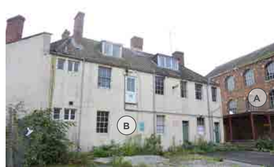
View of the North Elevation Facing into the Yard
