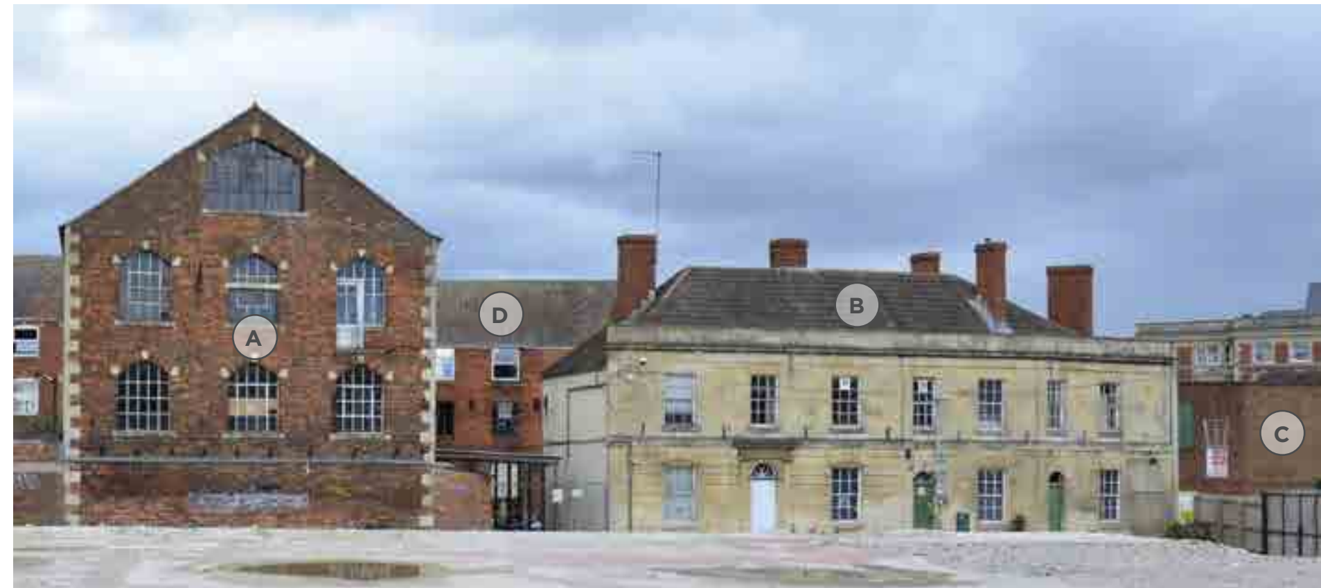
View of the South Elevation Facing the Railway
