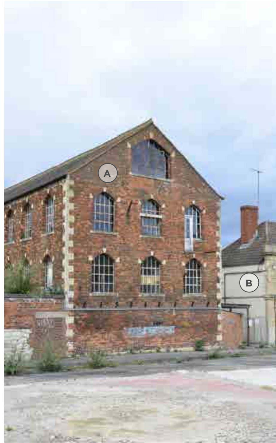
View of the South Elevation Facing the Railway
