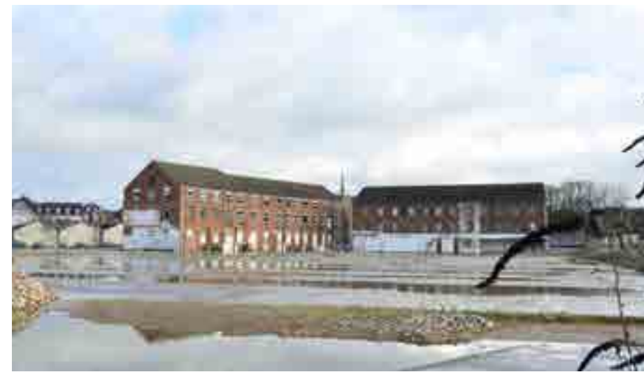
7 View of Innox Mill and the former Cloth Factory
