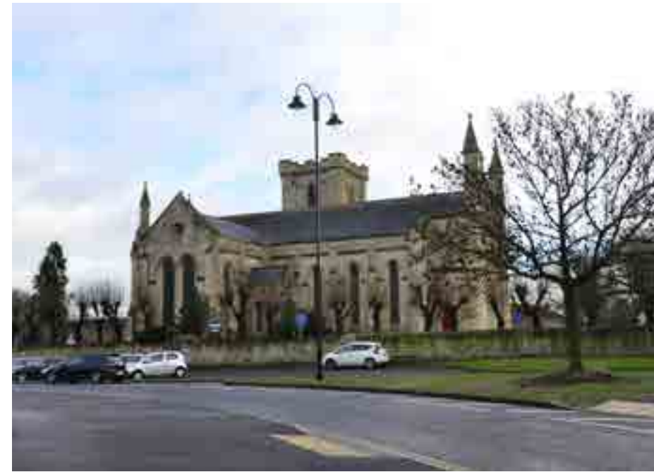
View of Holy Trinity Church situated on island site surrounded by the A363
