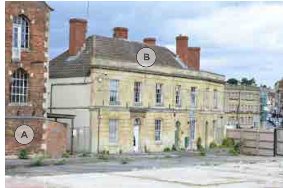
Innex Place viewed from within the site. The view looks up Wicker Hill and Fore Street.
