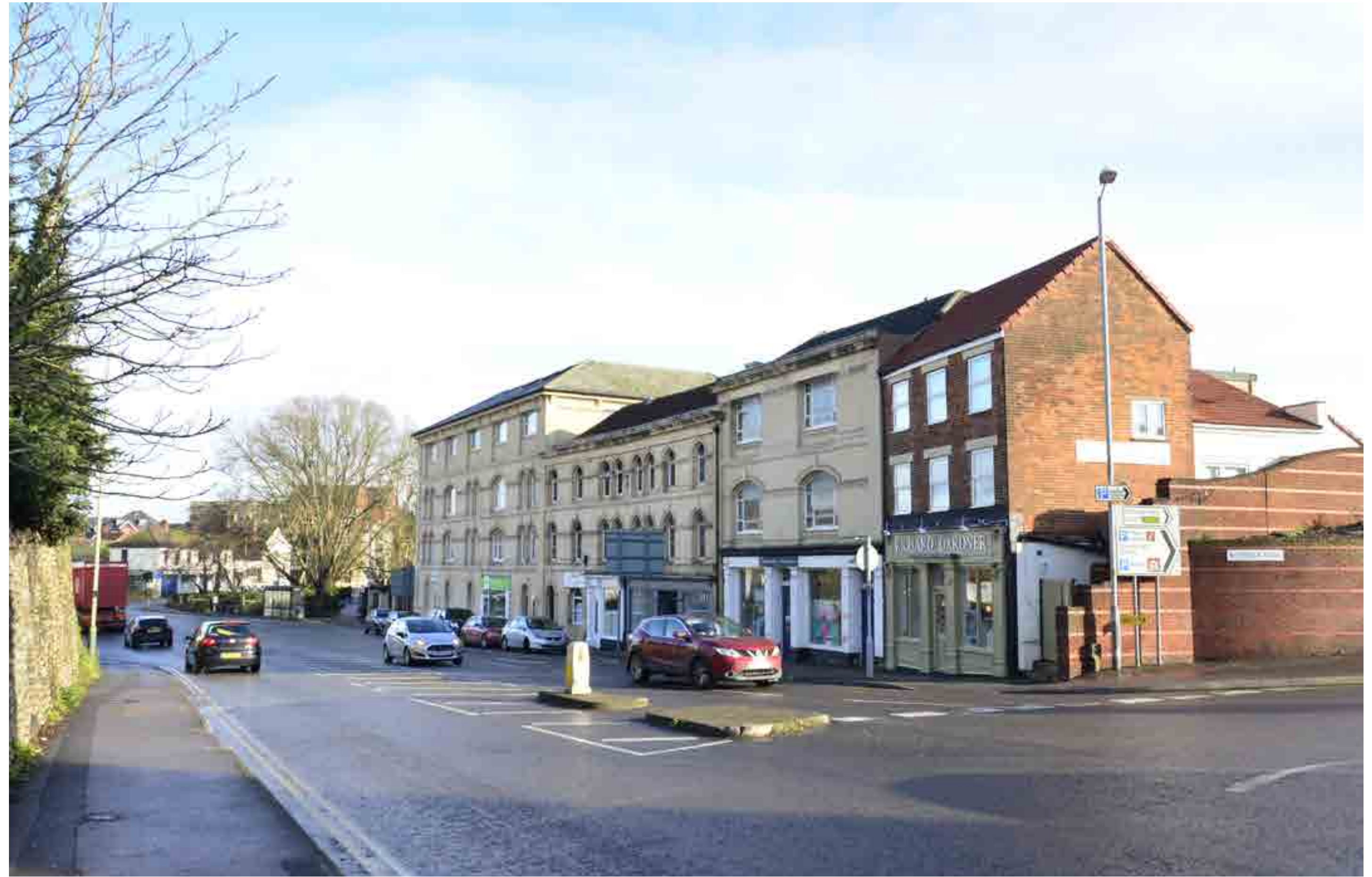
Buildings along Stallard Street looking northeast
